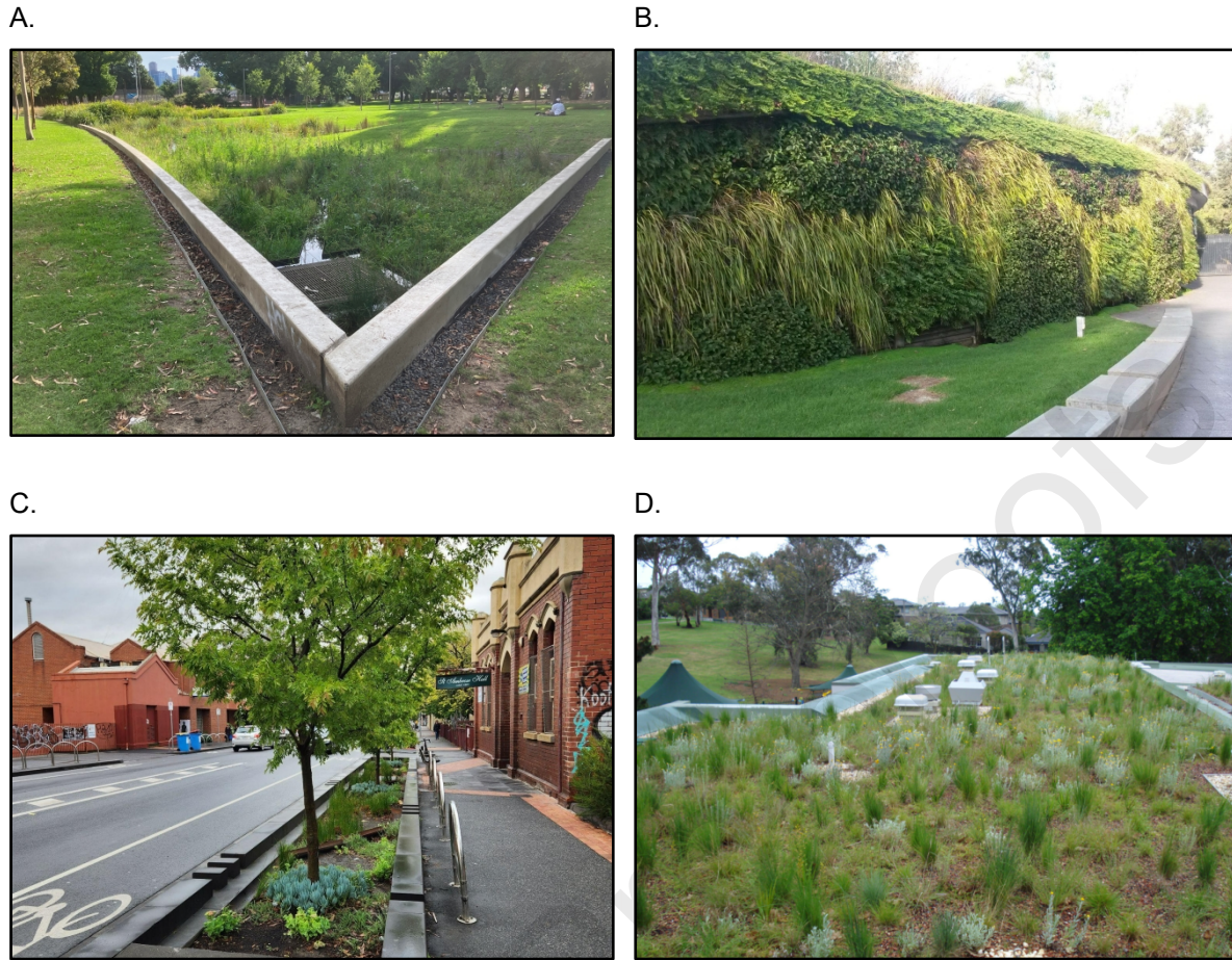
Figure 3. Urban green spaces at the WSUD technology scale. (a) Bioretention basin in Edinburgh Gardens, Melbourne: the system treats up to 24 ML of runoff per year, supplementing irrigation of sports ovals in the park; (b) Curved green wall project at Adelaide Zoo in South Australia: this vertical greening system is irrigated with harvested stormwater and excess water drains into a bioswale (Water Sensitive SA, 2015); (c) Street tree pit in Melbourne with passively irrigated trees; (d) Green roof in Minifie Park Early Childhood Centre, Melbourne. The green roof was planted to enhance biodiversity. Photo credit: University of Melbourne. All photos were taken by authors or credited to owner with expressed permission for use.
