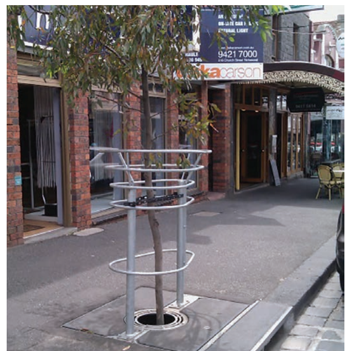
Figure 18: Smith St. biofiltration systems
